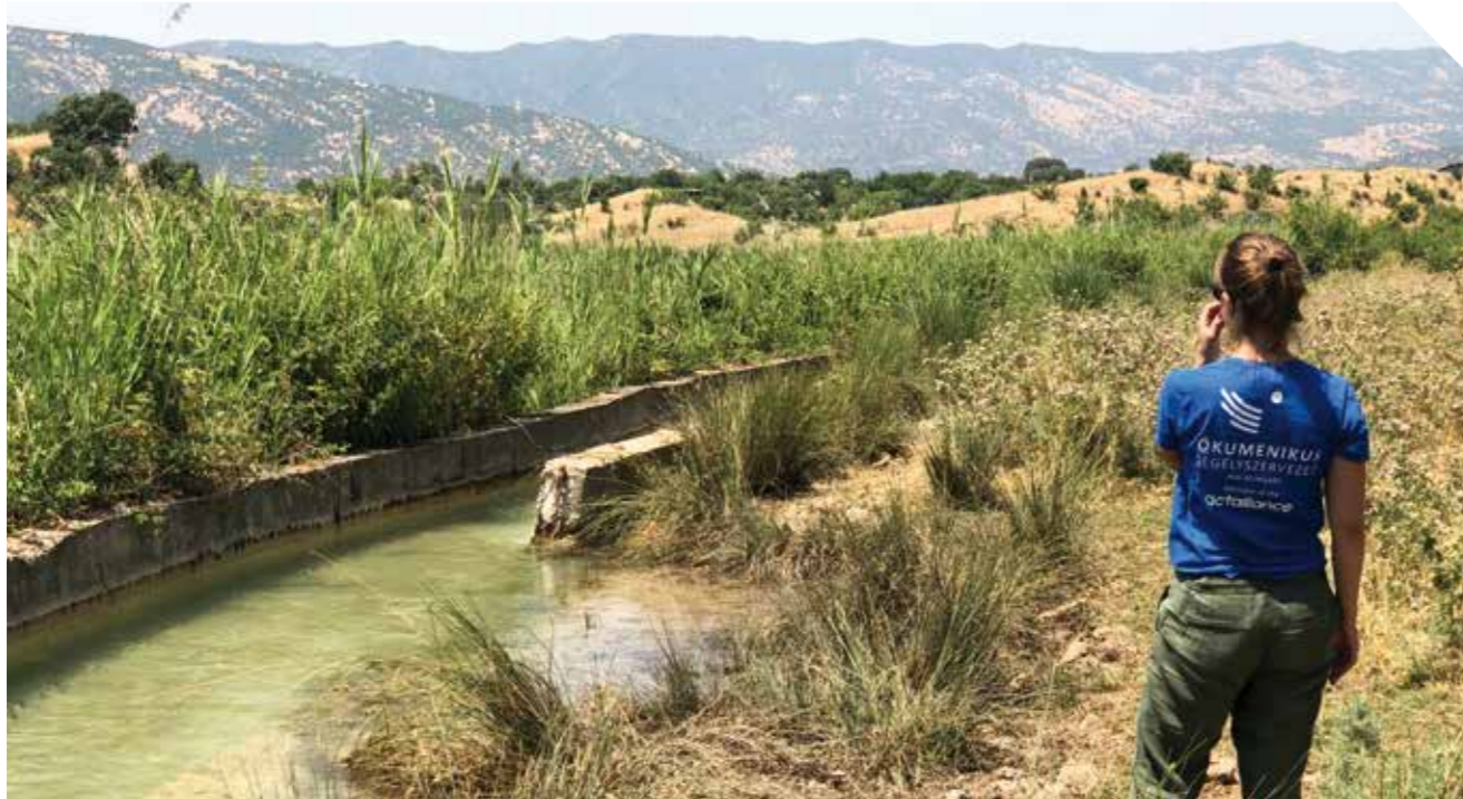
Reconstructed irrigation tunnel in Nahla Valley, Iraq Source: Hungarian Interchurch Aid
