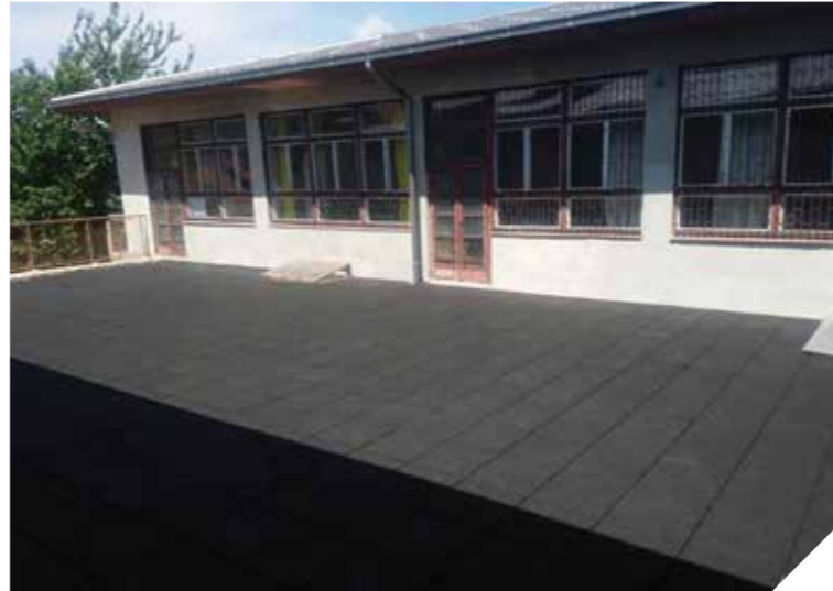
Renovated school in Bosnia and Herzegovina, implemented within the framework of a V4+Japan development cooperation program Source: Ministry of Foreign Affairs and Trade of Hungary
